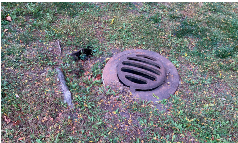
Drainage and erosion issue on west side of park
