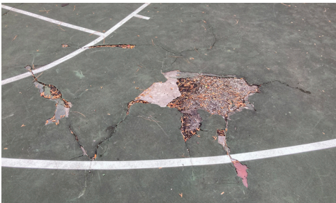
Spalling concrete at basketball court
